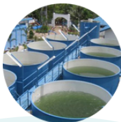
WTP/WWTP/ WATER SUPPLY
