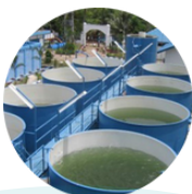
WTP/WWTP/ WATER SUPPLY
